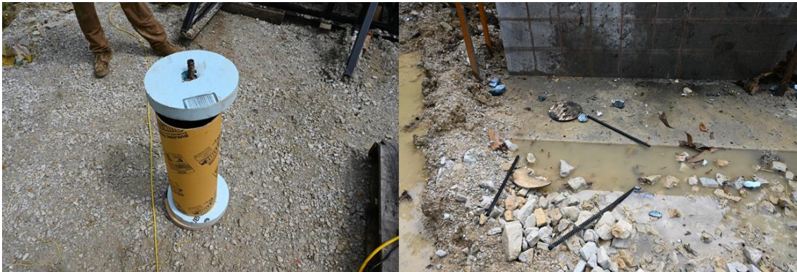
Figure A.63. Roof bolts
