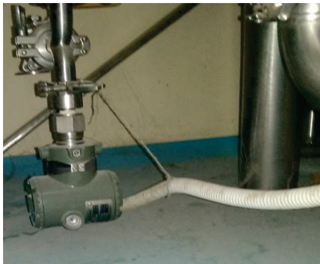
Gambar 2.2 Displacement Pressure Level Transmitter
