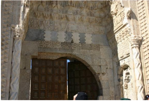
Figure 3. The Flat Camber Arch and The Inscription
