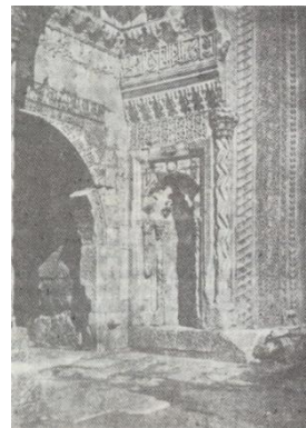
Figure 2. Sultan Han Portal 19 century (Y.Önge's archive)
