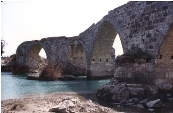
Figure 10. Overview of the Bridge
