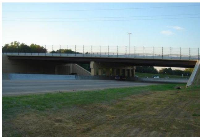
Figure 2. Pacific Street and interstate 680 highway bridge in Omaha, Nebraska
