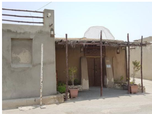
Figure 6. Using bracing in walls and wood in skeleton of canopies for relative resistance against earthquake
