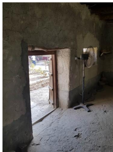
Figure 7. Using wooden frame of doors for resistance of walls, protecting thick walls with high thermal capacity causing suitable insulation of inside spaces
