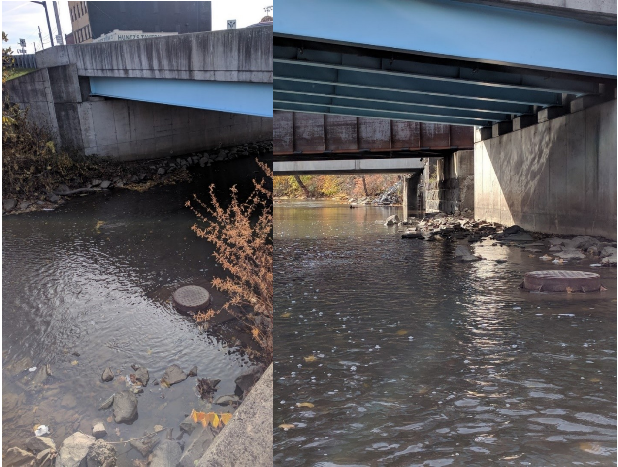
Figure 40. Sewer line manhole covers in Pine Creek at low flow situations.
