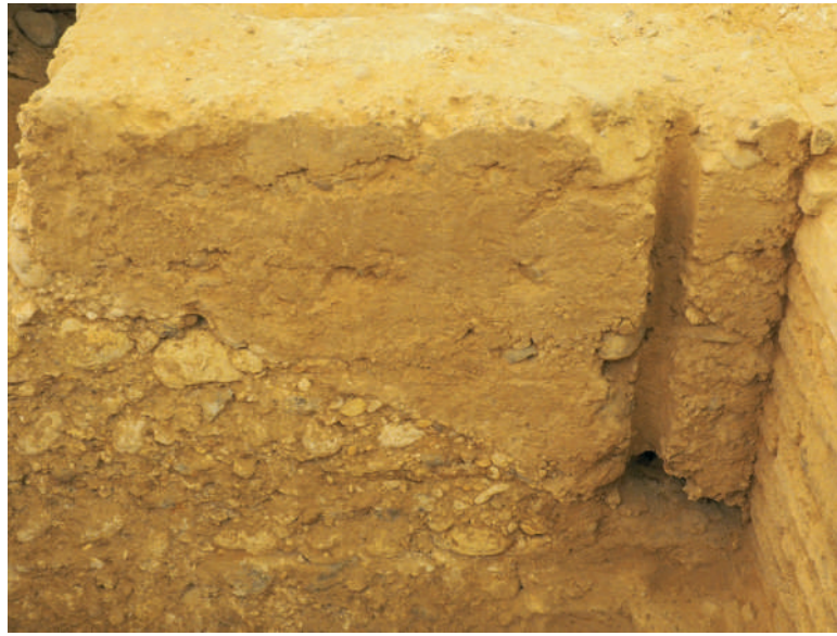
Figure 9. Ruins of the fence wall (exploration 1). Source: authors
