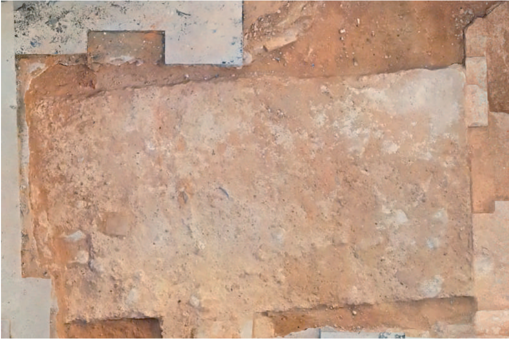
Figure 17. Lateral wall of the 13 th century bell tower, the bottom of which used the buttress of the diaphragm arch to close the structure (exploration 1). Source: authors
