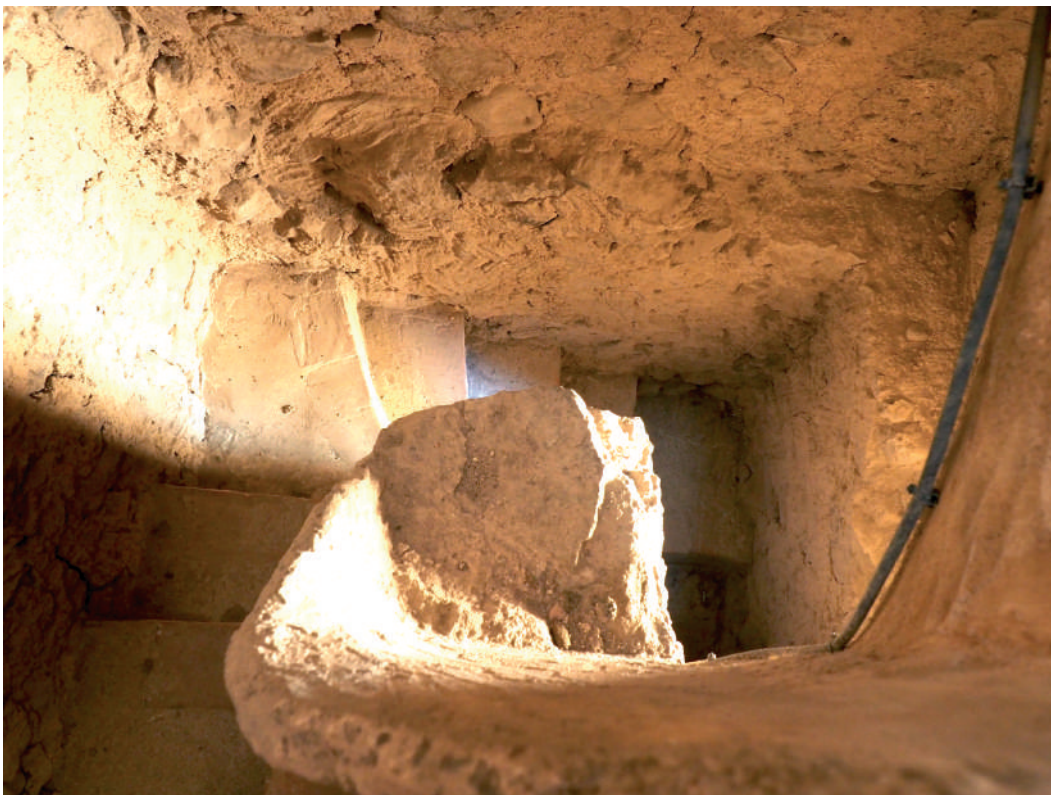
Figure 18. Lateral wall of the 13 th century bell tower, the bottom of which used the buttress of the diaphragm arch to close the structure (exploration 1). Source: authors
