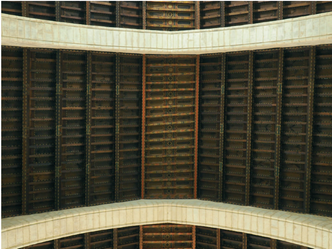
Figure 13. Roofing church San Pedro, Xàtiva. Source: authors
