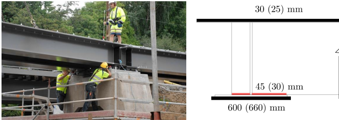
Figure 14. The railway bridge (during construction). Original flange dimensions and the dimensions after HFMI treatment in parenthesis. Red lines indicate HFMI-treated areas.
