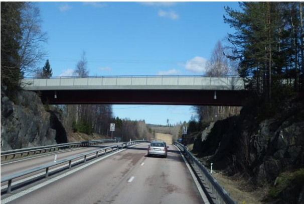
Figure 15. The simply supported road bridge.
