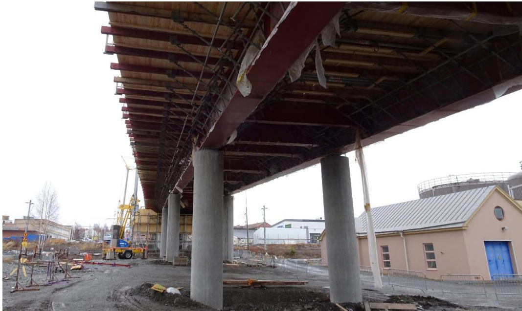
Figure 16. The continuous road bridge (during construction).
