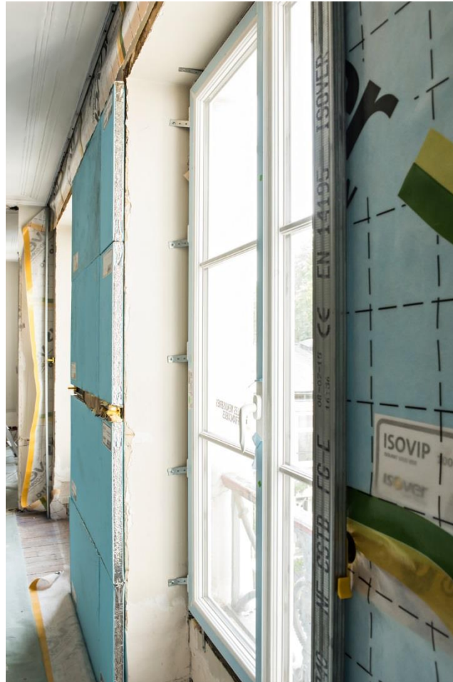
Figure 62 : OPTIMA-VIP system from ISOVER (Saint-Gobain) installed for internal retrofitting.
