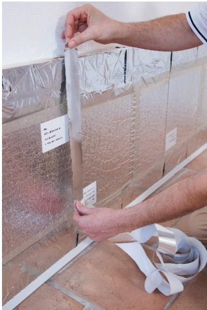
Figure 68 : Installation of the SLIMISOL system
