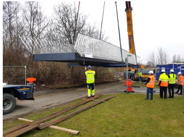
Figure 10. Installation of the bridge, Photo courtesy of Composite Design
