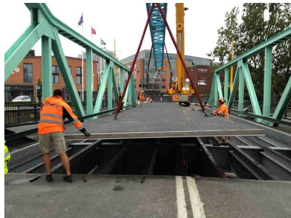
Figure 6. Installation of FRP deck panels, Photo courtesy of Per Andersson
