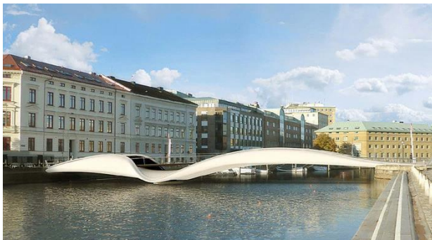
Figure 1. Concept of Kaponjär FRP bridge over Rosenlundskanal in Gothenburg. Picture courtesy of Ramböll
