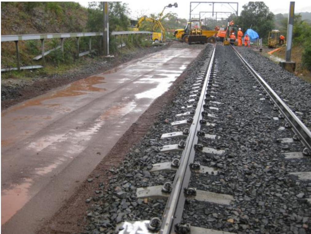
Figure 1. A typical ballasted track. The capping layer or called ‘subballast’ is prepared by compacting roller prior to laying ballast. In reality, the capping layer and subgrade are non-homogenous and cannot be accurately modelled by a simple constant elastic half-space nor a continuous layer. These layers are thus designed under higher safety margin or higher factor of safety by the allowable stress design concept [16-17]. The design takes into account the accumulated strains of these layers, which are often limited over a target design period (e.g. 15-25 years). Track maintenance cost function of deteriorated ballasted tracks will increase over years.
