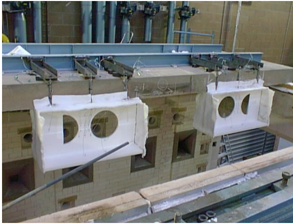
a) Attachment of beams to the soffit of chamber
