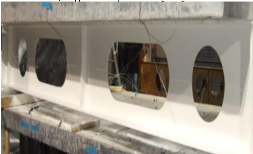
c) Application of intumescent coating along the beam
