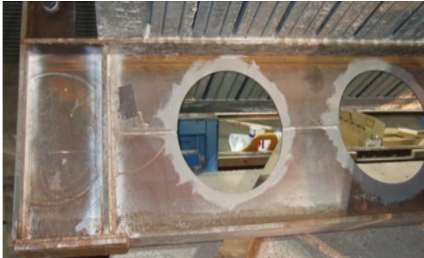
a) Application of primer coating around openings
