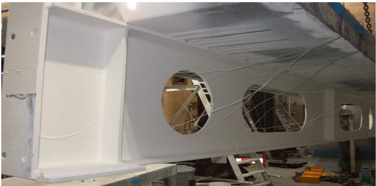
Figure 6.2-7 Thermocouples on protected CCBs
