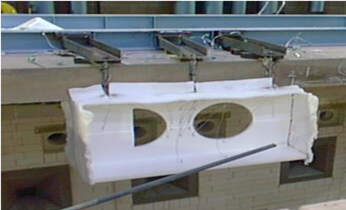
a) Connections of beams to the chamber using studs
