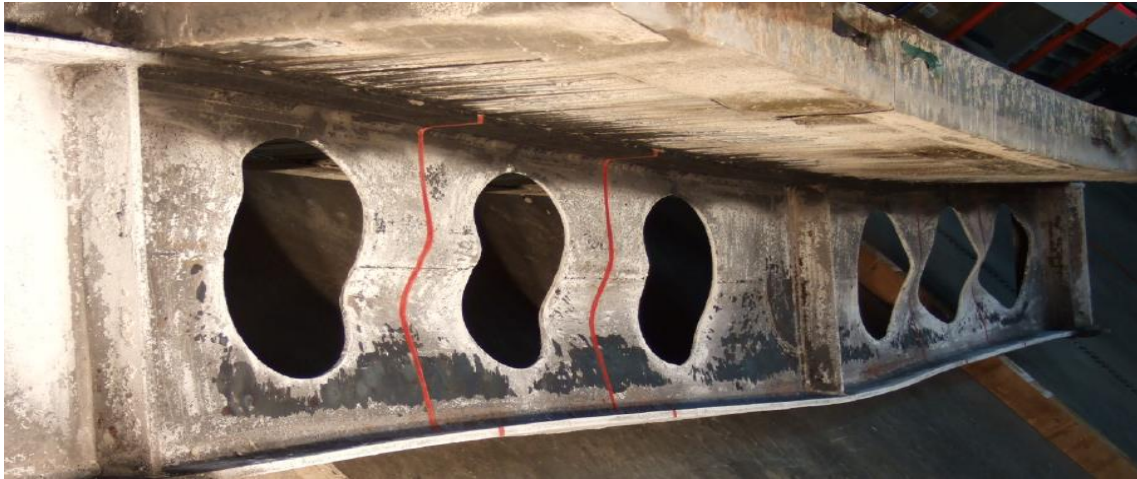
a) Deformed Beam 3, experiment
