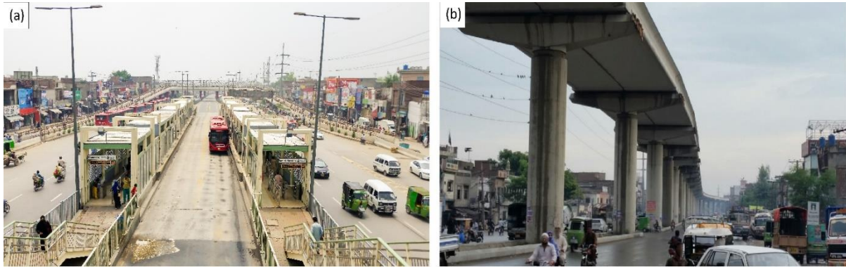
Figure 5. (a) Metro bus station showing rapid bus transit system, and (b) an elevated railway track for upcoming Orange Line for train in Lahore. Photographs taken on: 13 th July, 2017 and 30 th August, 2017 respectively
