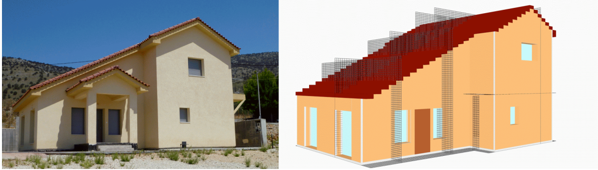
Figure 1. External photograph (left) and general computational grid (right) of the simulated building.
