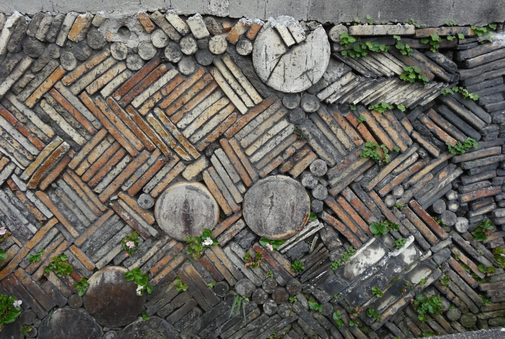
Kiln furniture (supports, sagars & shelves) incorporated into revetments around Seto, especially on the 'The Path of the Kiln Fence' (窯垣の小径).
