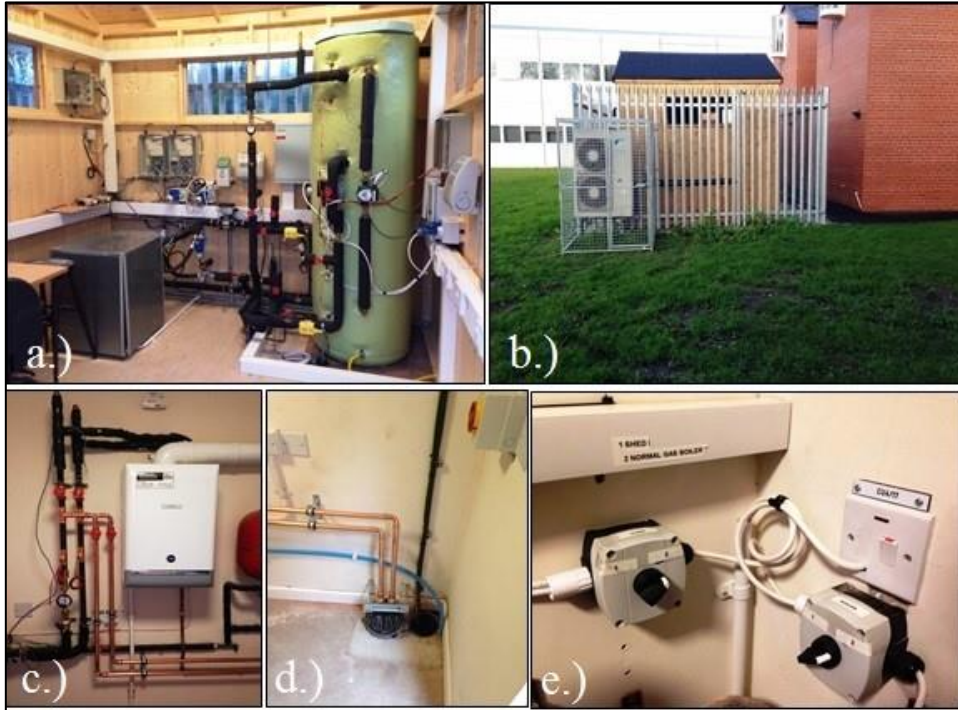
Figure 3 Field trial set-up: a.) Shed: Cascade heat pump indoor unit with R134a & 600l hot water storage tank, b.) Cascade heat pump outdoor unit with R410A, c,d,e.) modification in boiler room
