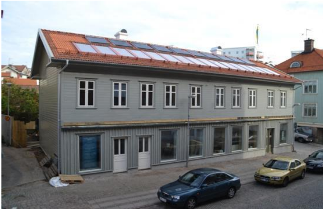
Figure 1 Solar panels on roof of Renovated building (© Lars Pettersson, Scandinavian Homes Ireland Ltd)
