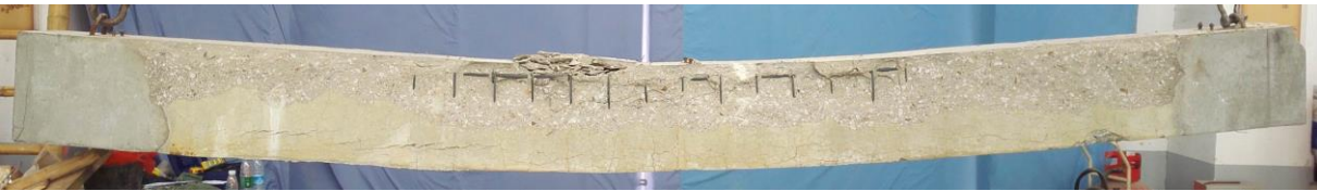
Fig. 4. Failure mode of the SRC beam
