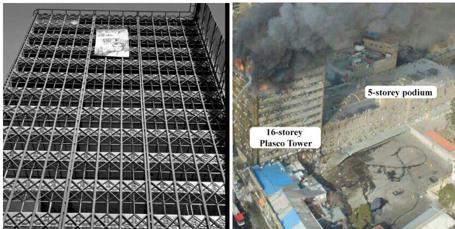
Fig. 1. Steel frame and bracing system around all sides of the Plasco tower; (b) the attached 5-storey shopping centre; (all images courtesy of IRNA)
