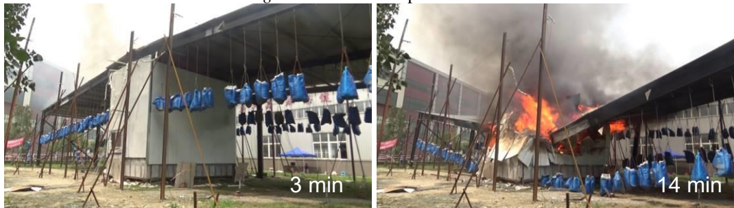
Fig.5. Structural collapse in Test 2
