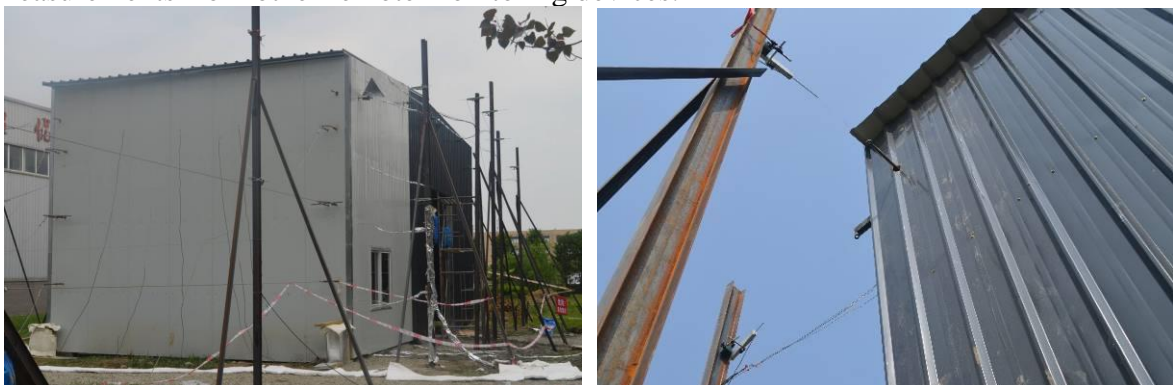
Fig.3. Mounting of LVDT on the structure
