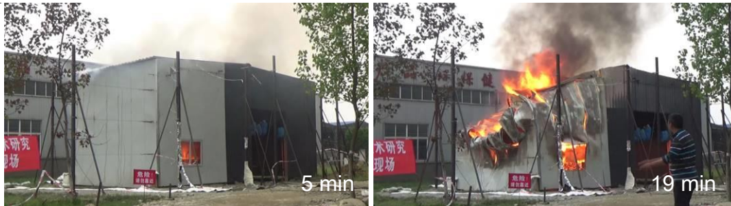
Fig.4. Structural collapse in Test 1
