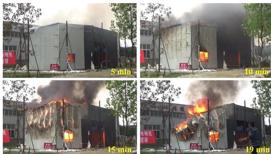
Fig. 8. Collapse process of the steel structure
