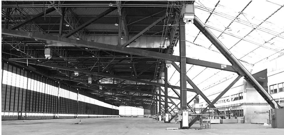
Figure 1: The hangar HN6
