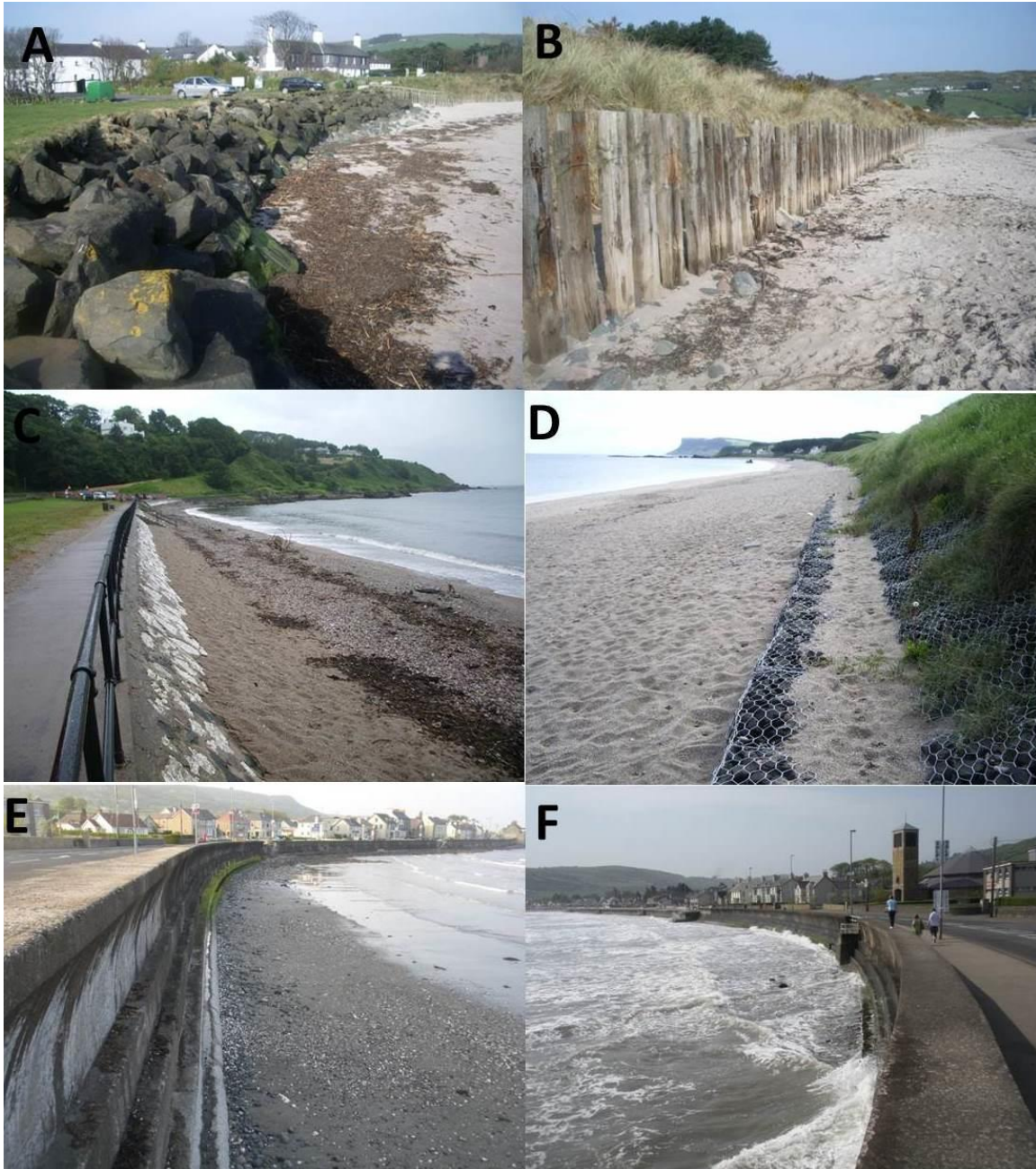
Figure 5. A. Cushendun rock armouring at a car park. B. Railway sleepers used as sea defence, Cushendun. C. Sloping stone wall, Cushendall. Gabbion baskets, Red Bay. E. and F. Near vertical, stepped seawall at Carnlough at low and high tide.
