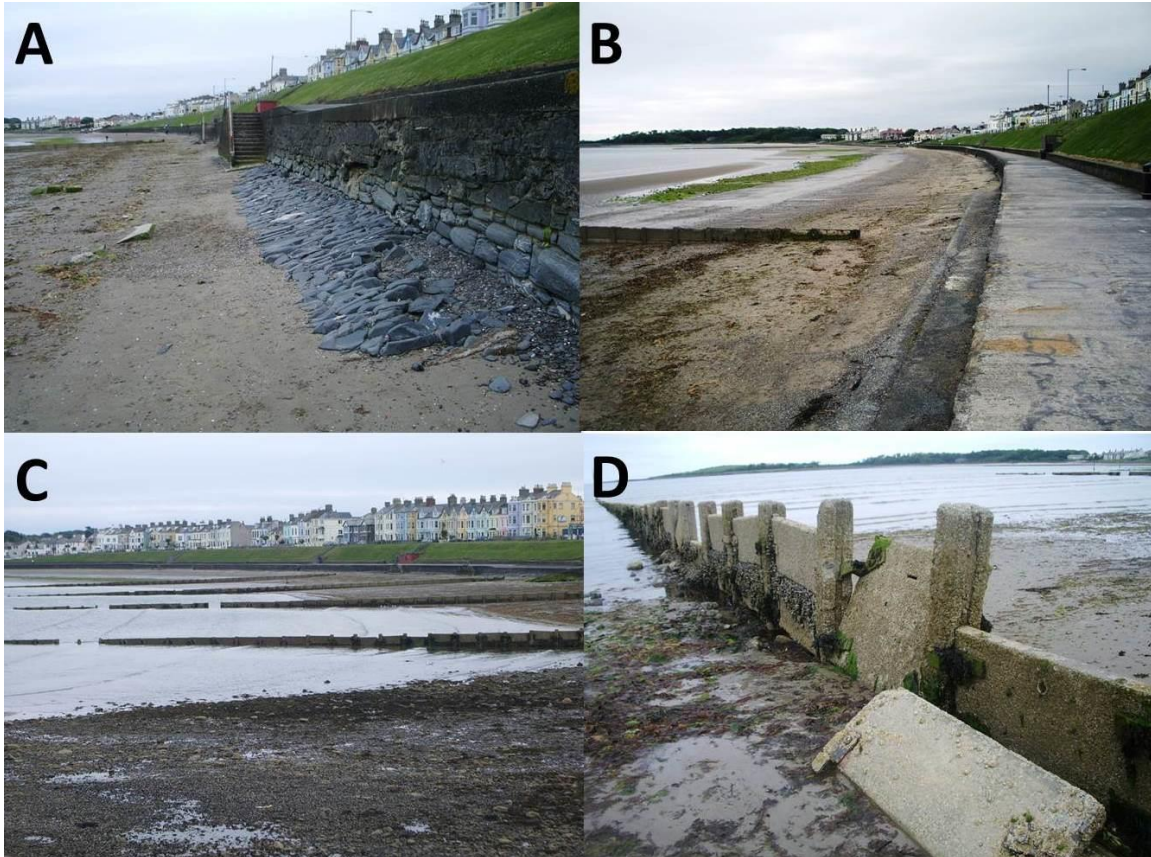
Figure 8. Ballyholme, Bangor. A. Sea wall and subsequent toe defence. B. Low promenade and seawall. C/ Groynefield/ D. Collapsing concrete groynes
