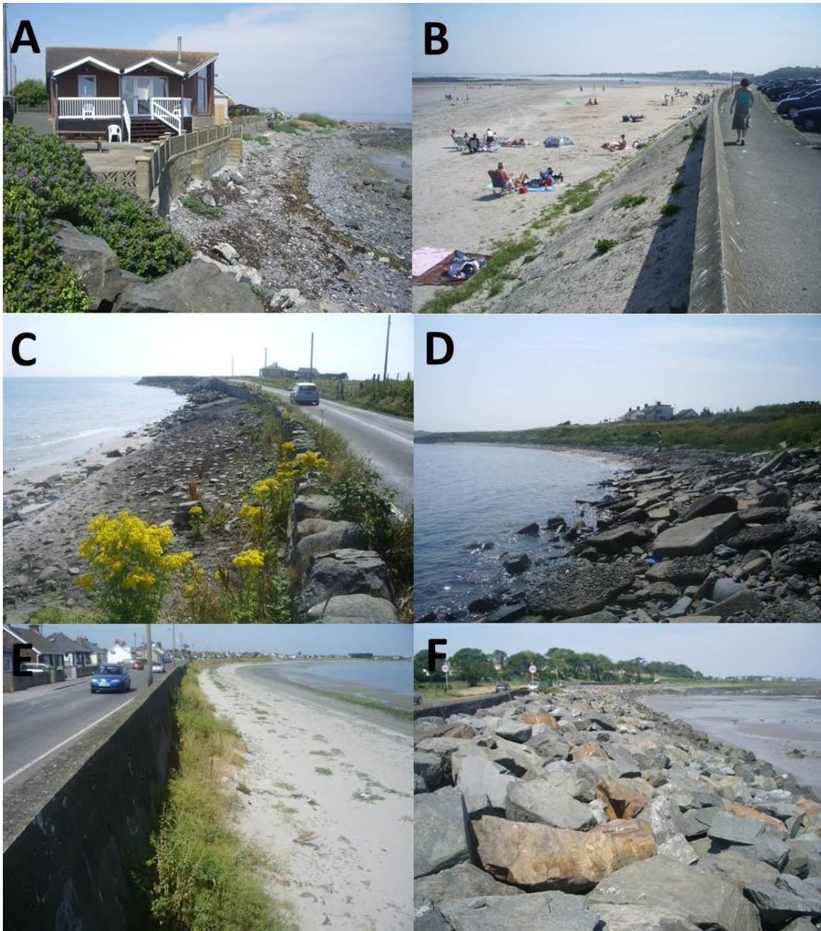
Figure 7. Sea defences on the outer Ards Peninsula. A. wall and rock armour defending house. B. concrete wall defending car park. C. Concrete wall defending road. D. Rubble dumped as sea defence. E. Vertical wall defending road. F. Massive rock armour defending road.
