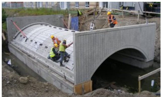
Figure 12b. Completed arch bridge before covering with backfill.
