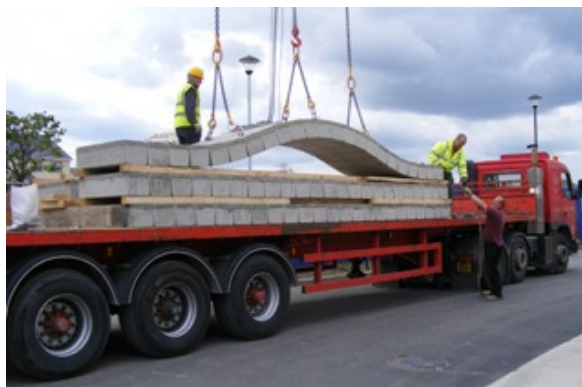
Figure 12a. Flat pack "Flexiarch" system brought to site
