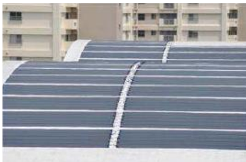
Figure 5. Global Solar – Roof with flexible CIGS laminate
