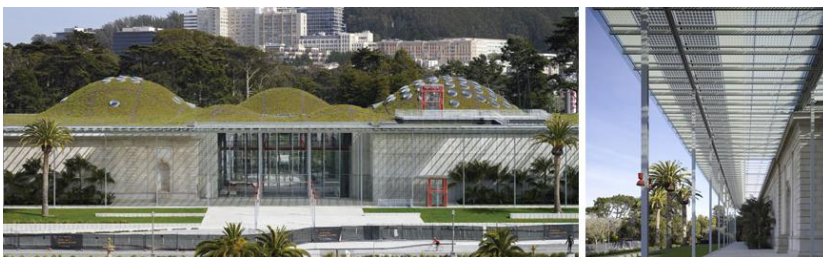
Figure 6. View of the Academy and the circumferential canopy with the photovoltaic cells [Available online from www.calacademy.org , www.dezeen.com (accessed November 2014)].
