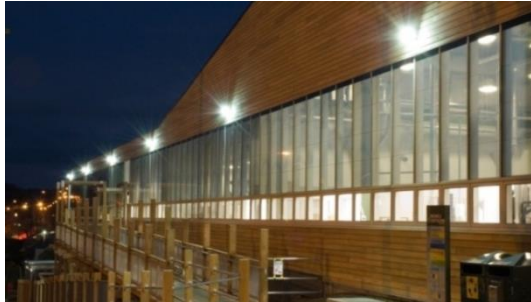
Figure 7. View of northern facade, consisted of photovoltaic glazing [Available online from www.mcoldowiepartners.com.au (accessed November 2014)]
