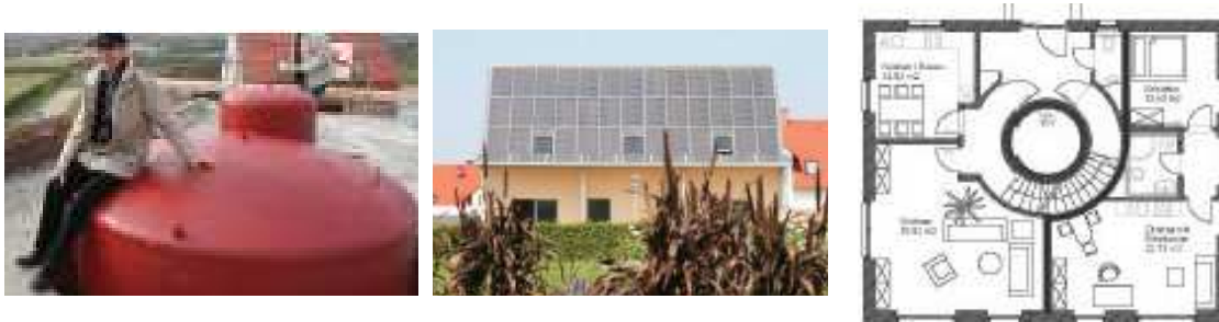
607 Figure 19. Solar water tank integrated in a solar building in Regensburg [52].
