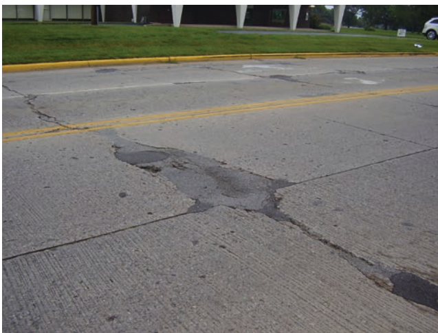
FIGURE 3 Patched concrete joint spalls (Source: R. McDaniel).
