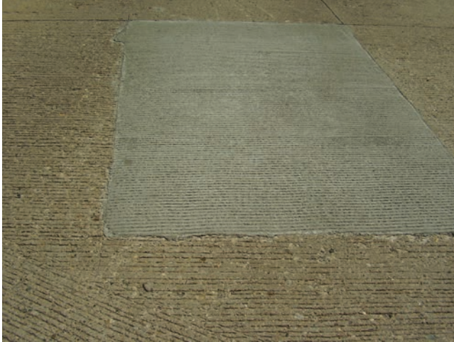
FIGURE 12 A sawed patch on concrete pavement with reinstated tining (Source: R. McDaniel).
