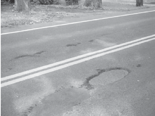
FIGURE 2 Delamination of surface layer (Source: CLRP).
