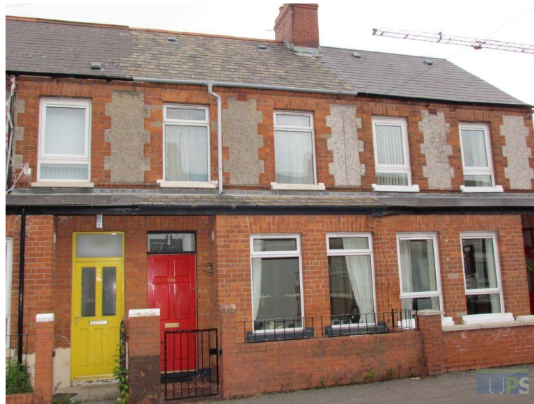
Figure 2.2. Typical Green Street homes
