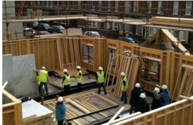
Figure 2.7. The Green Street properties under construction
