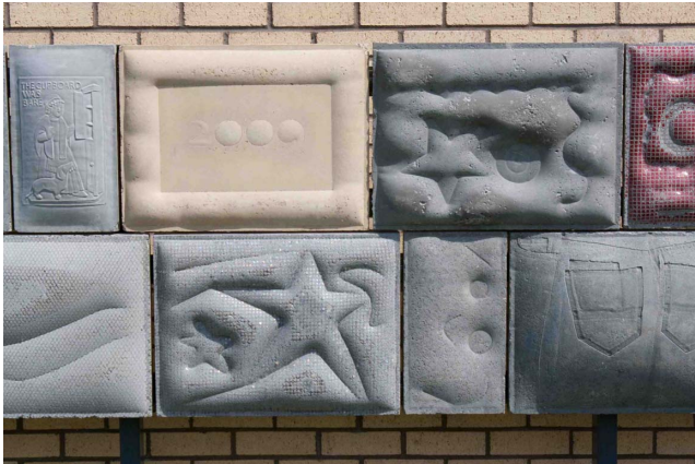
Figure 3. Formwork panels with range of surface finishes
