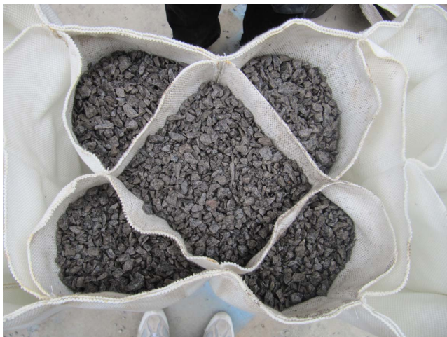
Figure 9. Cavity construction formwork
