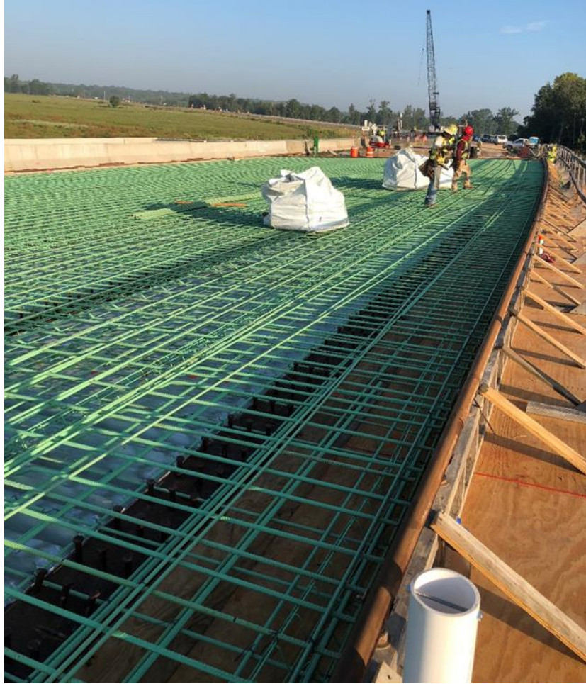
Figure 17. Site view from bent 1 looking to bent 2.
