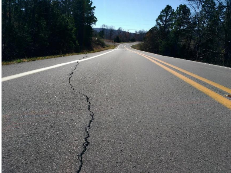
Figure 3- Longitudinal Crack Located on Highway 7 (Used with Permission from Salman Rahimi)
