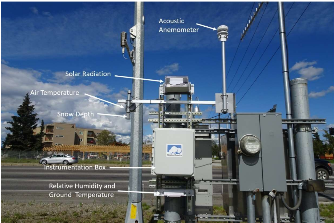
Figure 2 Cowles Street installation
