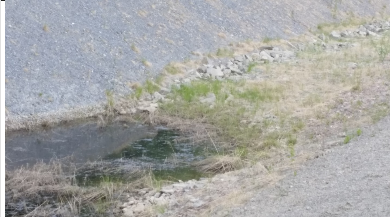
Figure 1.3 Dalton Hwy., MP 19, may be different project. Sparse clumps on slide slope, but vegetated in pond. Note erosion control by ditch lining with rocks.
