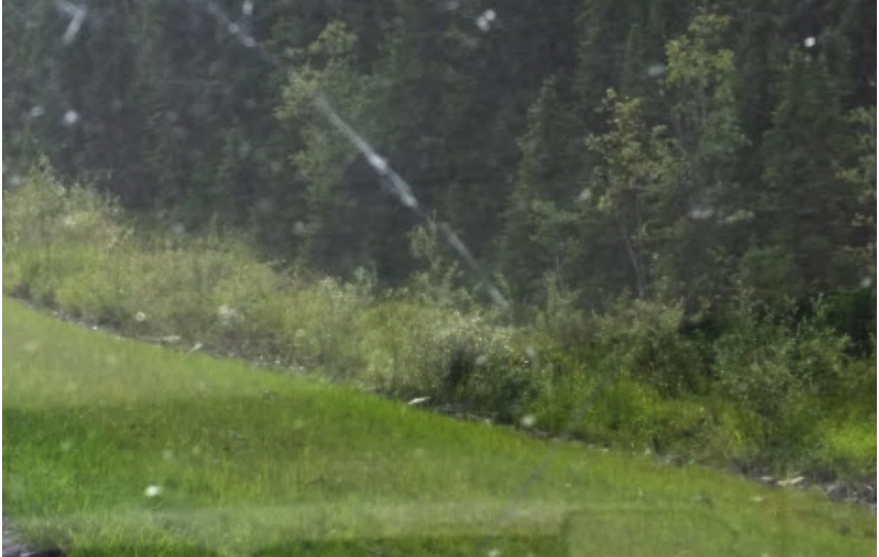
Figure 1.12a Example of grass in rills (tracks), about MP 109 Elliott Hwy.; recent project. Slope here is quite green. This is new revegetation from recent project. Note woody shrubs, probably from former road, and native trees in background.
