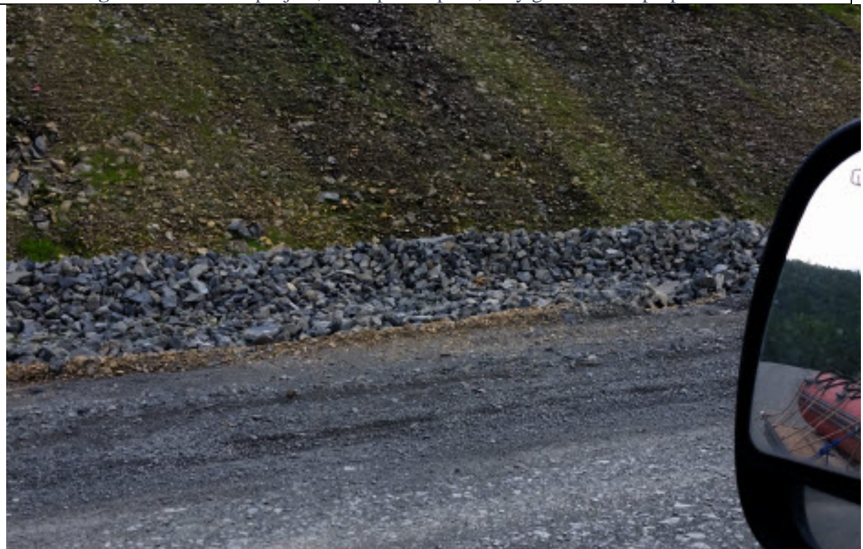
Figure 1.11b Riprap in ditch.
