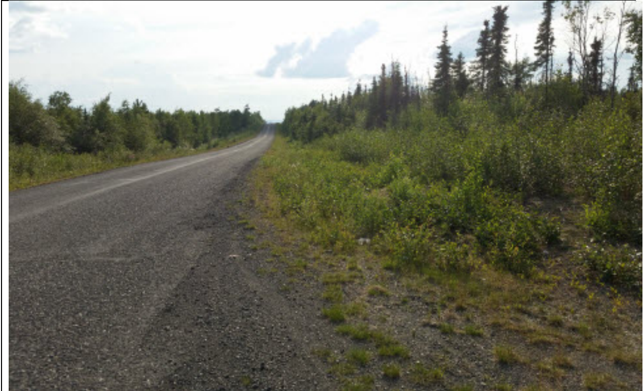
Figure 2.14 Example of an old project, MP 120–127 Elliott Hwy., probably 1994. Note the woody plants are sparse. This ROW has surely been cut down. Note contrast with taller plants on right. Some grass is evident.
