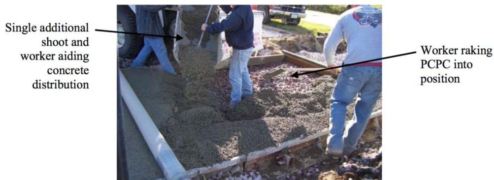
Figure 2.15 Pervious concrete placing (reprinted from Kevern et al. 2006)
