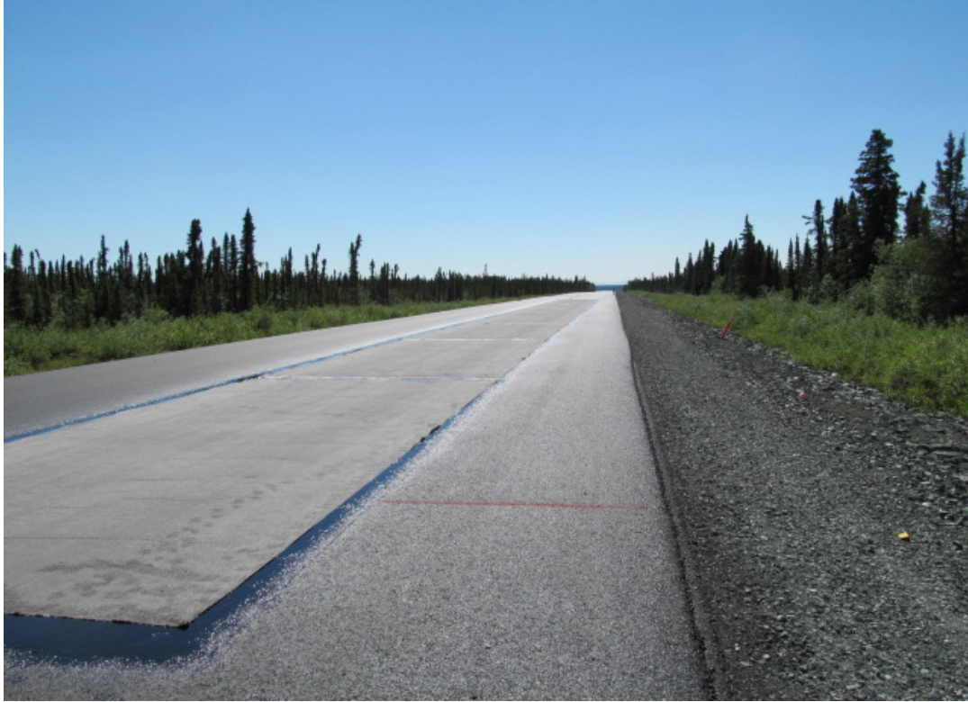
(a) Construction of the test section
