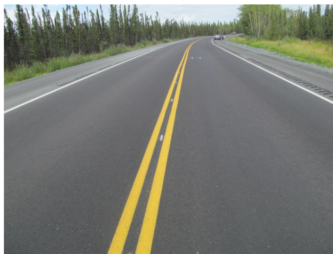
Figure 3.19 Control section (300 feet in area 4)
