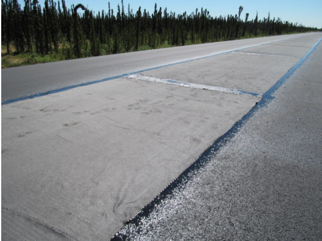
(a) Construction of the test section
