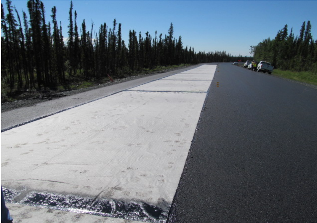
(a) Construction of the test section
