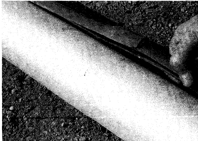
Figure 3.13 Thermistor string installed on the thermosyphon.
