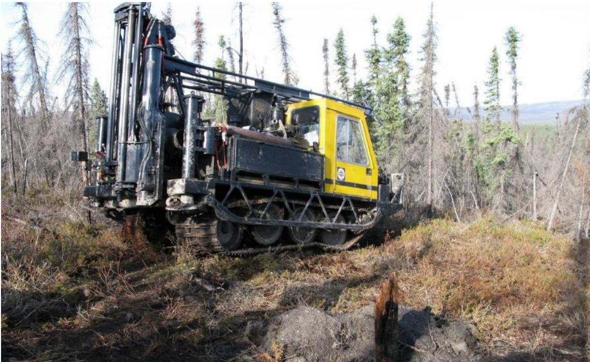
Figure 17. Drill rig at the Dalton Highway Innovation Project field site, May 2008
