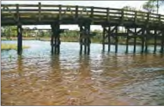
Horseshoe Bayou Bridge
