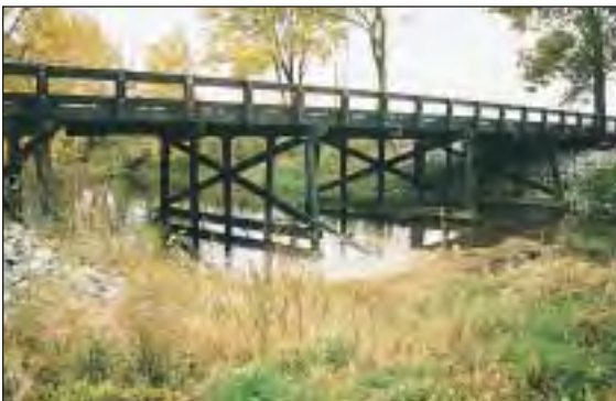
Pipe Creek Bridge
