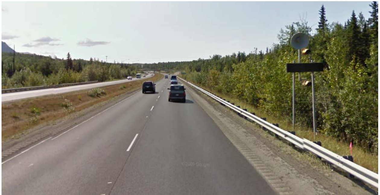
Figure 3. Southbound Freeway Mainline Blank Out Sign and Alarm Speaker (Source: Google Maps ©2011 Google)
