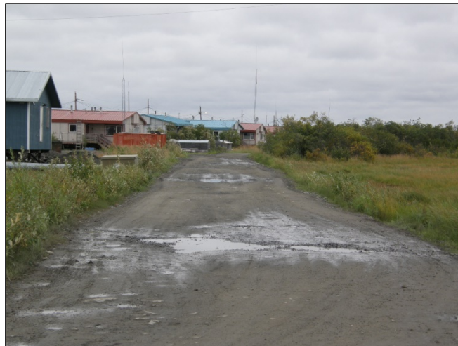
Figure 7. Improperly graded road resulting in poor drainage off of the road surface
