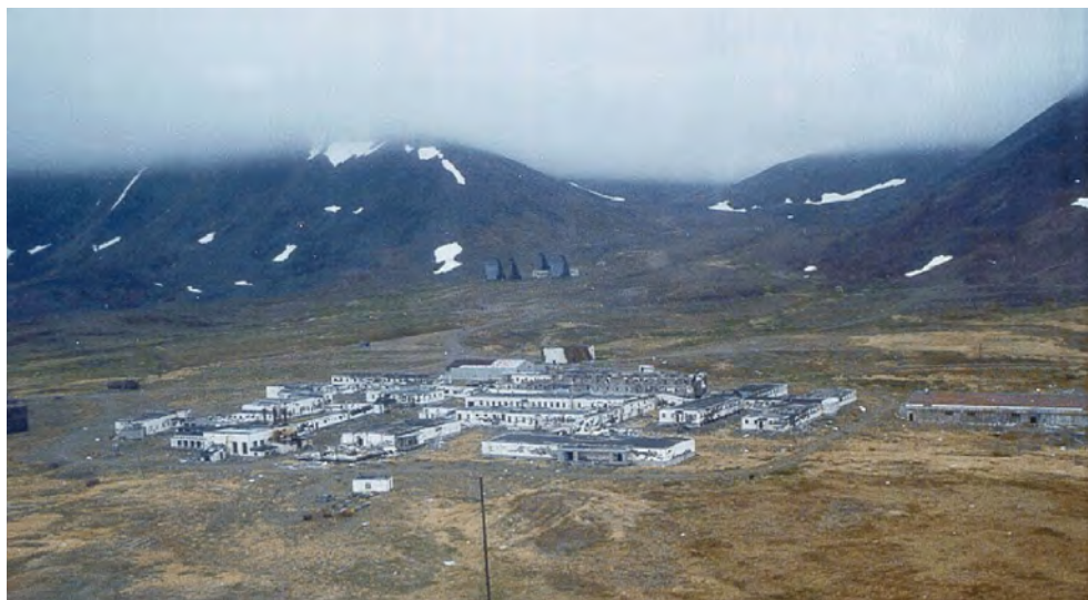
Aerial view of the former Northeast Cape Headquarters facility. The buildings were removed and disposed off-island in 2003. U.S. Army Corps of Engineers (n.d.) via Wikimedia Commons (21 Mar 2007).
