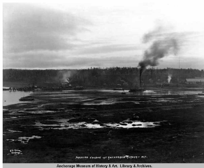
Figure 6: Alaska Engineering Commission Dredges Ship Creek, October 7, 1917.
