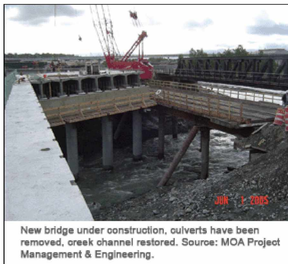
Figure 21: Construction of Bridge over Ship Creek, 2005.
