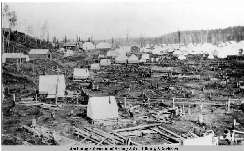
Figure 2: Clearing Land to Construct a Tent City on Ship Creek, Early Summer, 1915.
