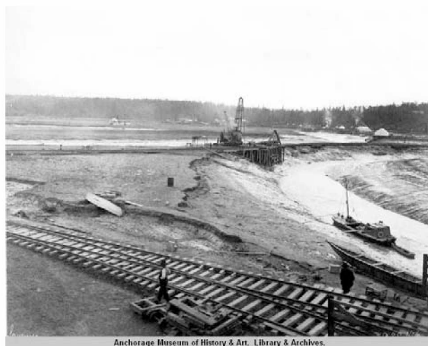
Figure 8: Railroad Bridge Construction, Ship Creek, 1915.
