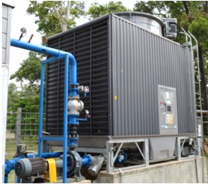
Fig. 2.7 Cooling tower
