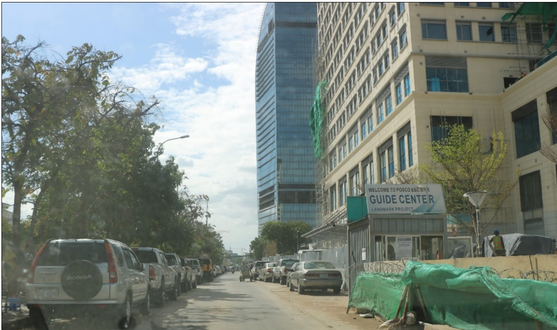
Fig.7.27 HSAs (road, under construction building, and the field along the road)
