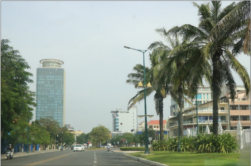
Fig.6.22 HSAs (buildings at the right side) in high-density area.
