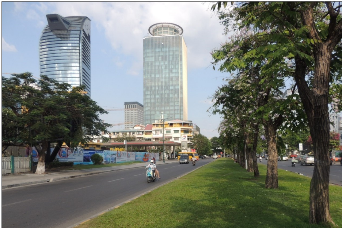
Fig.7.25 HSAs (gasoline station and buildings in front of it, left side)
