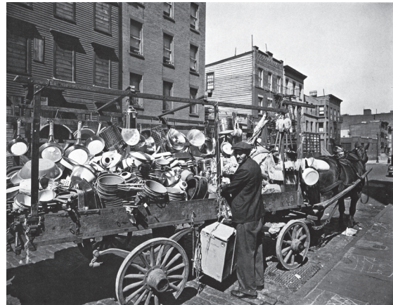
Figure 13 Berenice Abbott, "Traveling Tin Shop," Brooklyn, May 22, 1936.
