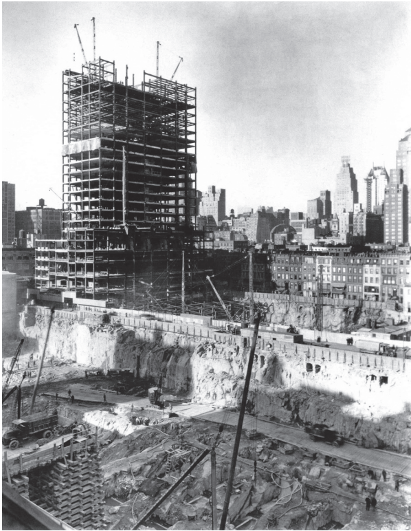
Figure 15 Berenice Abbott, "Excavation and Skelton of New Building," New York, circa 1930.
