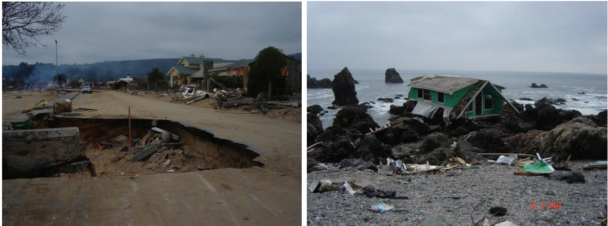
Figure 9. Effects of 2010 Chile Tsunami on Biobio Region. Left: Scour at the coastal street at Dichato town. Right: Wooden house washed away by the tsunami and deposited over rocks at Tumbes, inside the Bay of Concepcion.
