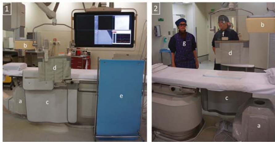
FIG. 4. Lead protection and staff position: 1:View from operating side; 2: View from non-operating side; (a) x-ray tube; (b) x-ray detector; (c) Table mounted lead drapes with extension panel; (d) Movable ceiling mounted lead glass shield with lead drapes; (e) Moveable stand-alone shield; (f) Common location for fluoroscopic operator; (g) Common location for scrub nurse.
