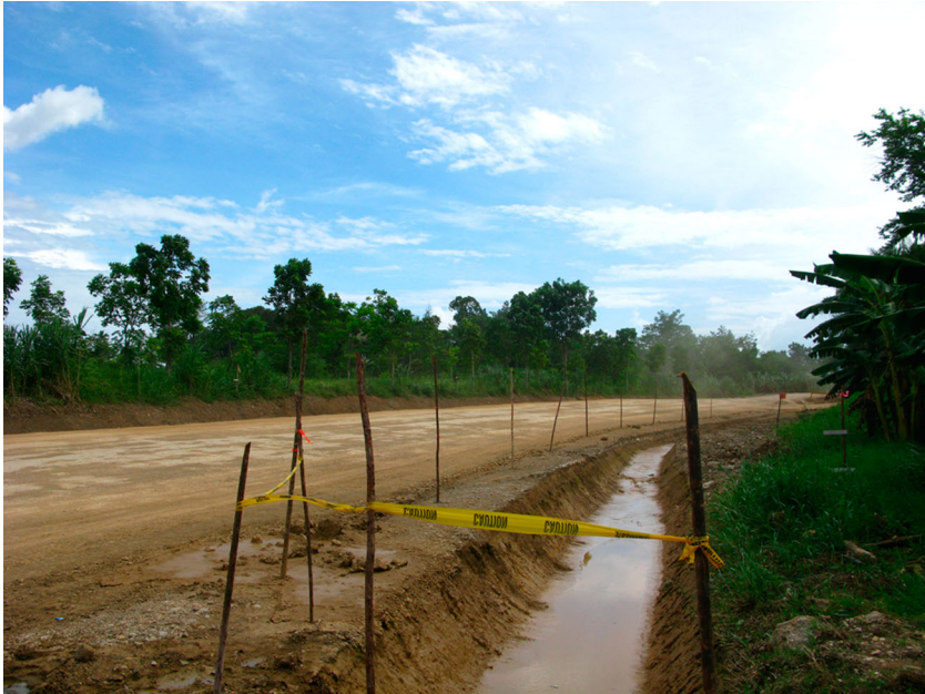
Figure 2. Works continue to complete the paving of the Southern Highway, 2009.
