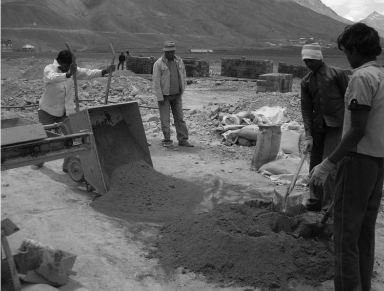
Plate 12.4 Making mud bricks on site
