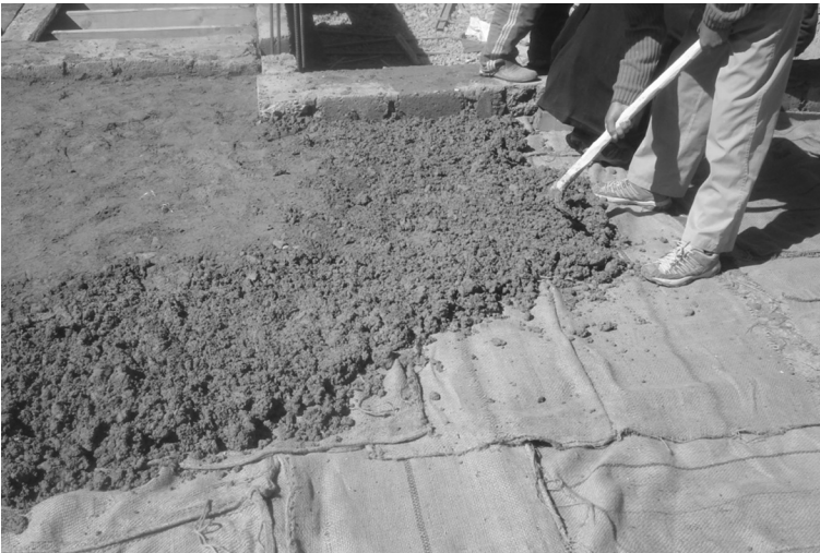
Plate 12.6 Flat mud roof
