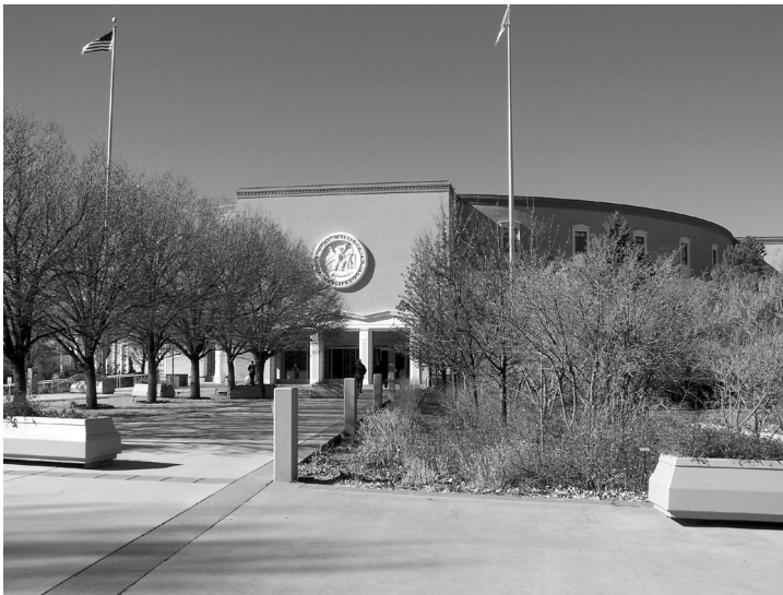
Plate 6.4 The New Mexico state capitol in Santa Fe
