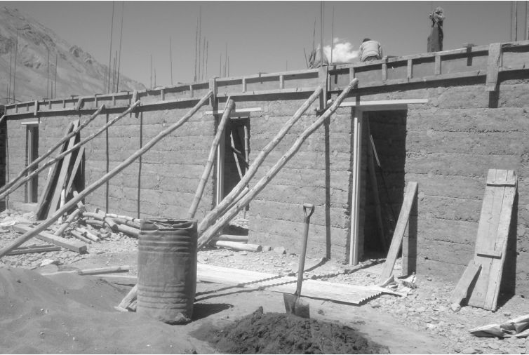
Plate 12.2 Rammed Earth Construction for walls
