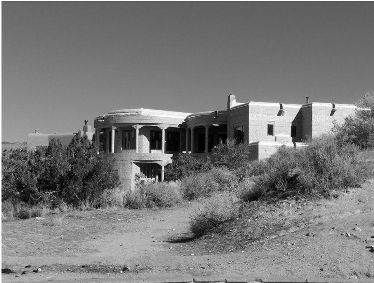
Plate 6.3 The Pueblo Revival/Santa Fe Style demasked – under the ‘adobe’ facade is the conventional two-by-four and plywood structure (new houses in Santa Fe)
