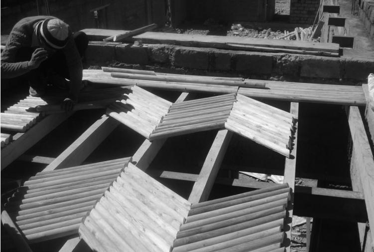
Plate 12.5 Recycled wood for formwork
