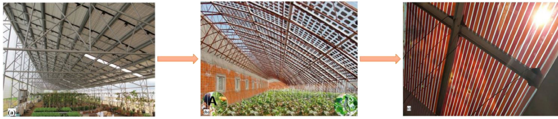
Fig. 1. Revolution of PV greenhouse (a) crystalline silicon modules greenhouse (Castellano et al., 2016), (b) thin film amorphous modules greenhouse (Hassanien et al., 2016) and (c) semi-transparent DSSC greenhouse.
