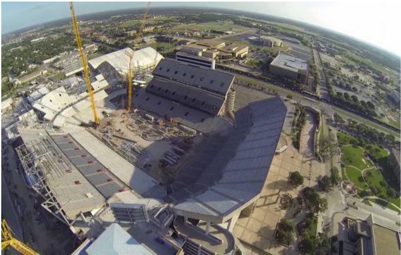
Figure 10. Kyle field renovation project 2014-2015
