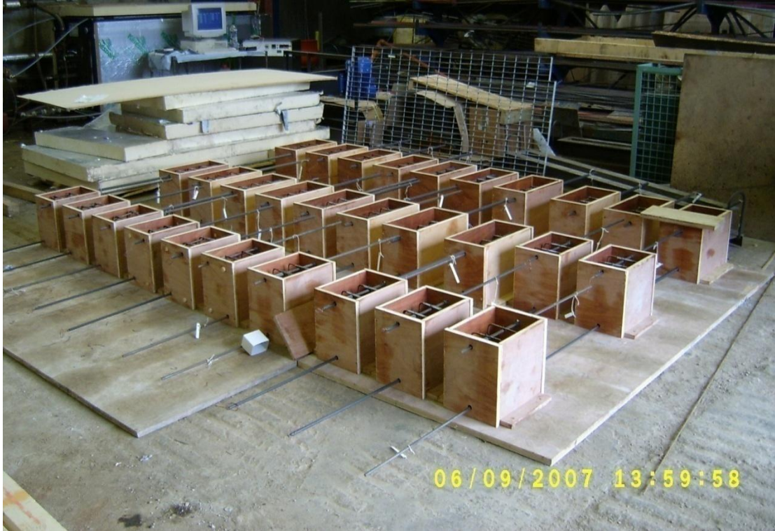
Figure 4.2: 30 beam end type specimens ready for concreting
