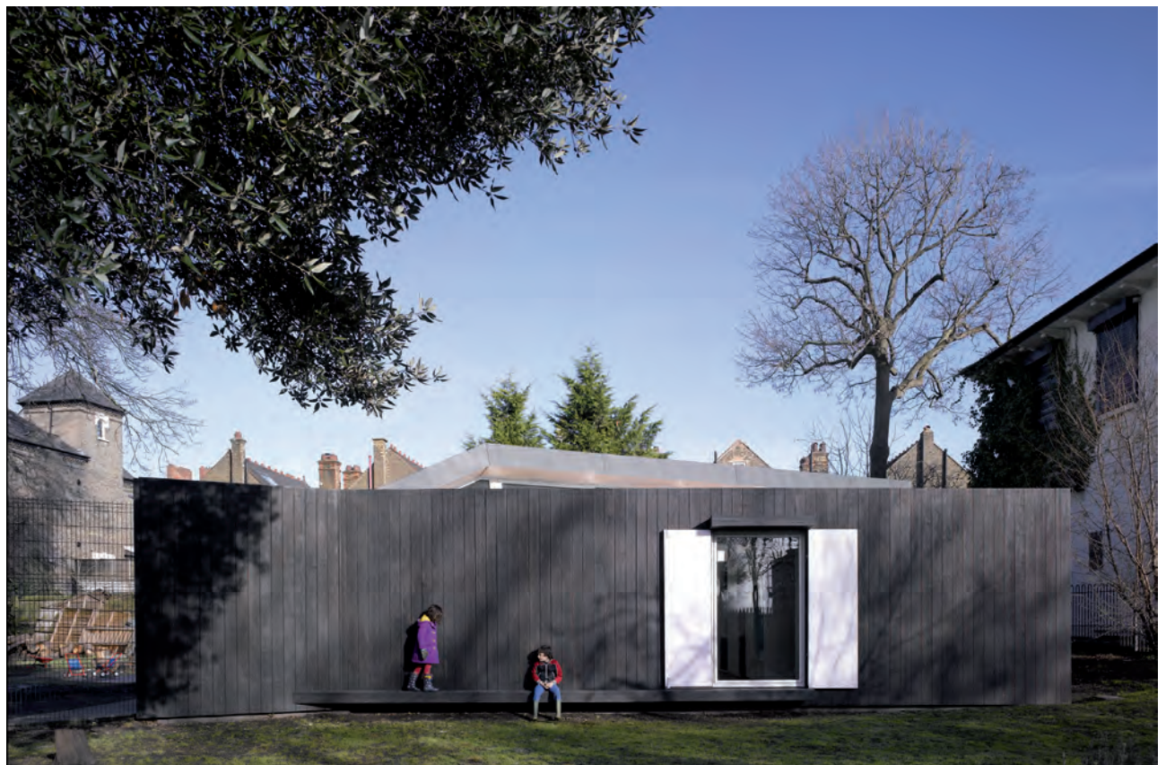
Fig. 06b External wall, door open, photograph Nick Kane
