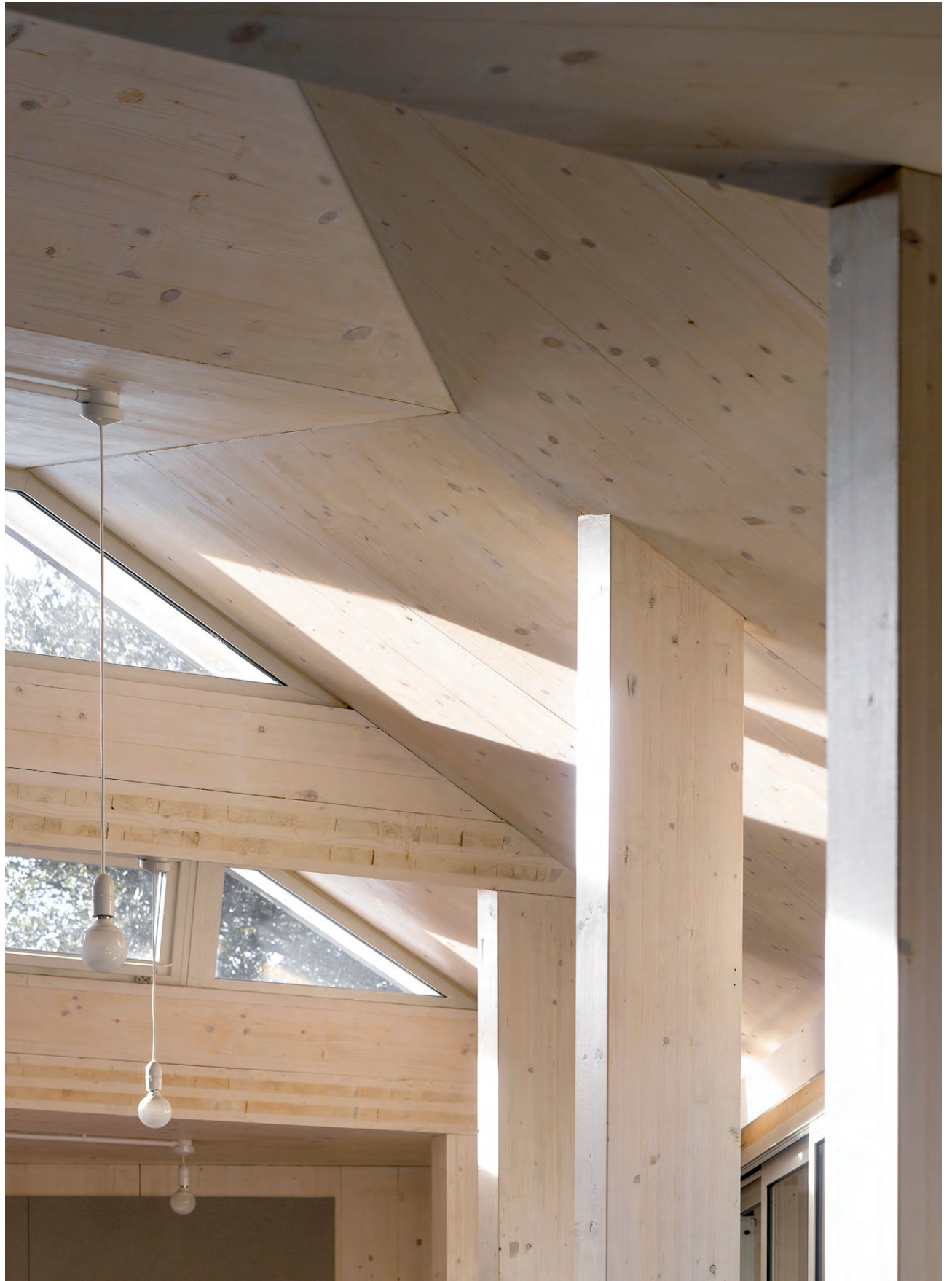
Fig. 17 Roof lights and ceiling, photograph Nick Kane
