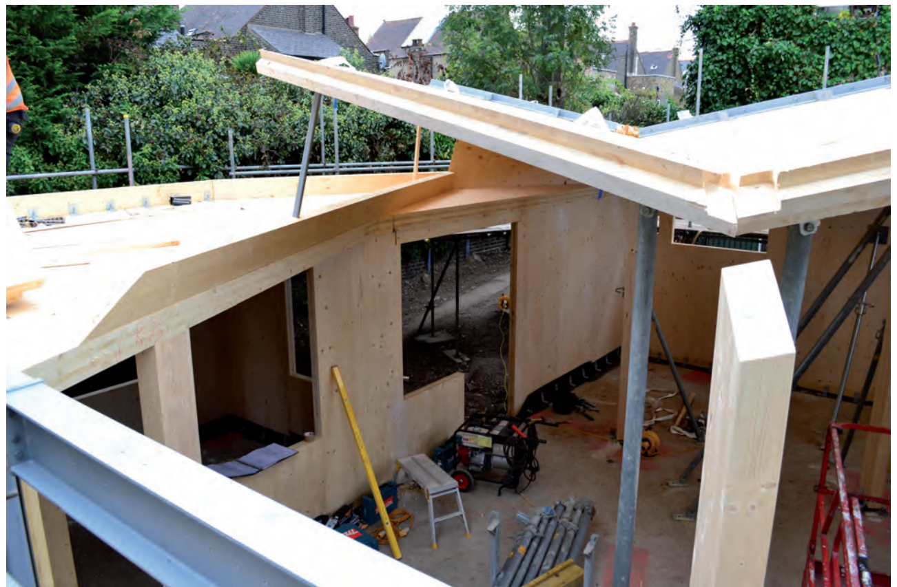
Fig. 11a 11b Building under construction
