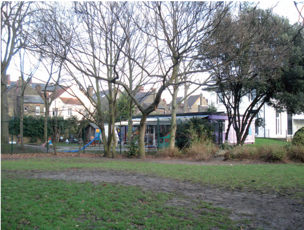
Fig. 02 Former nursery building
