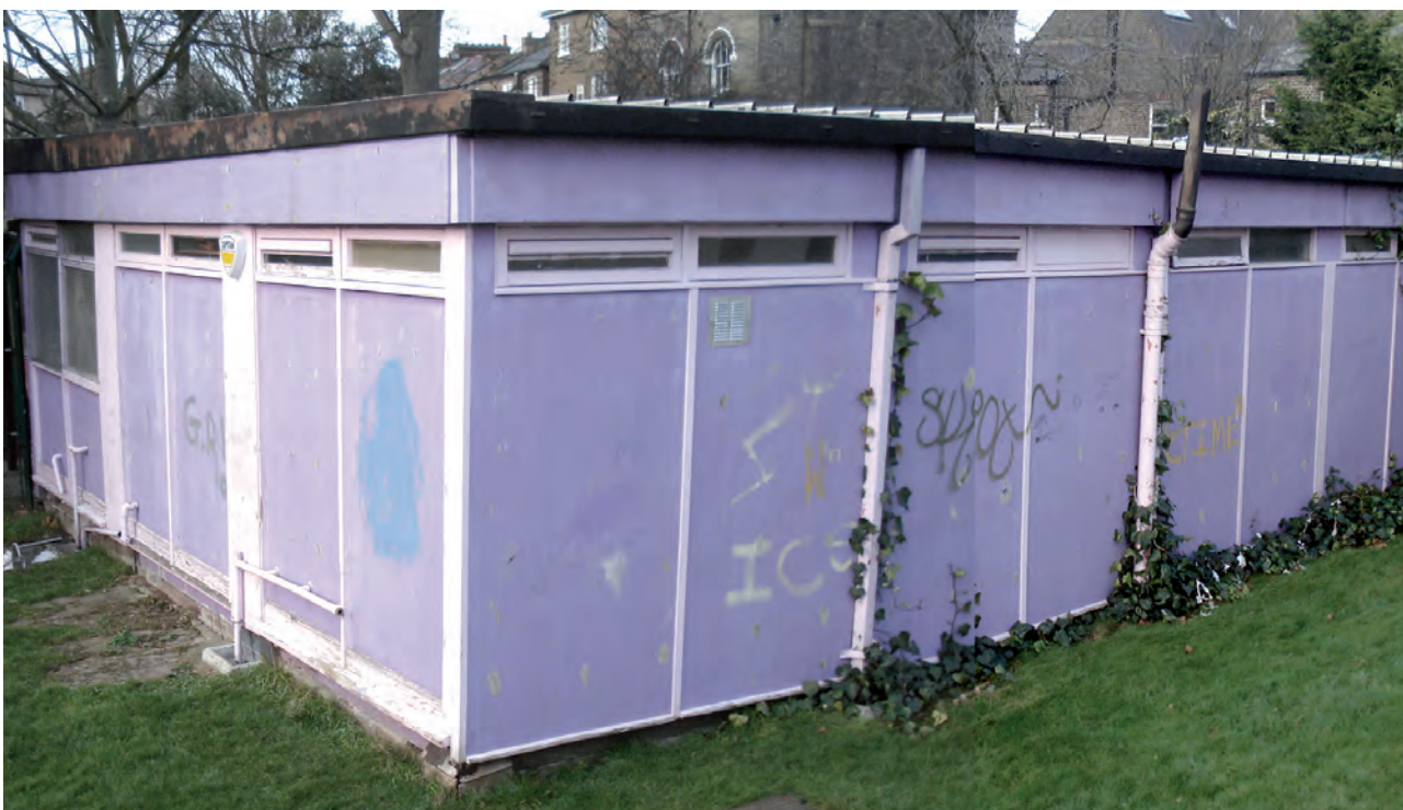
Fig. 03 Former nursery building
