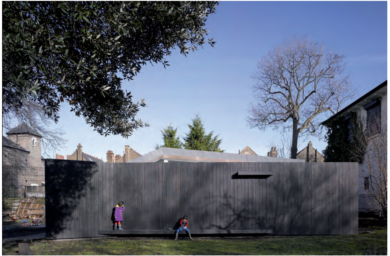
Fig. 06a External wall, door closed, photograph Nick Kane
