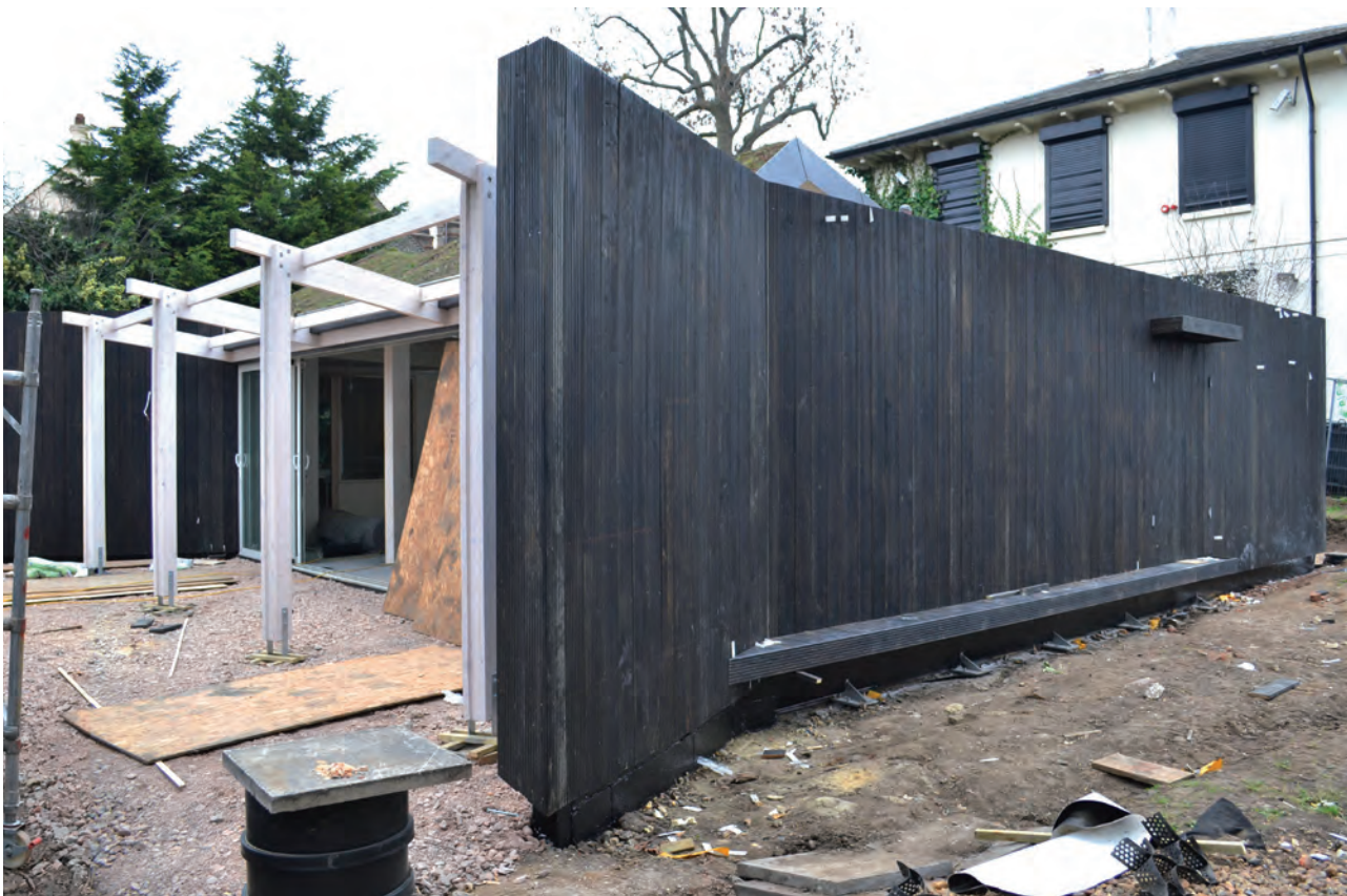
Fig. 13 Building under construction
