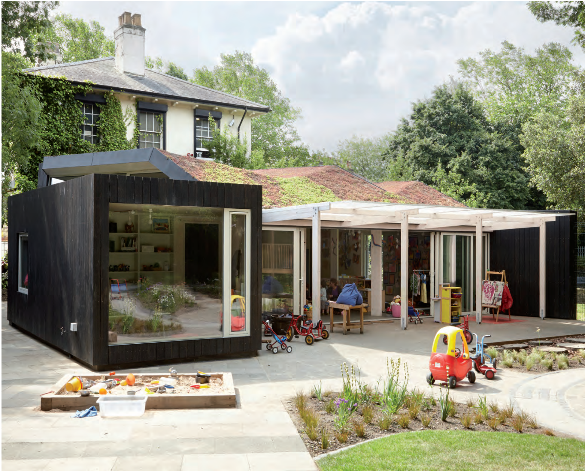
Fig. 35 Building – Garden Interface showing sedum blanket on roof
