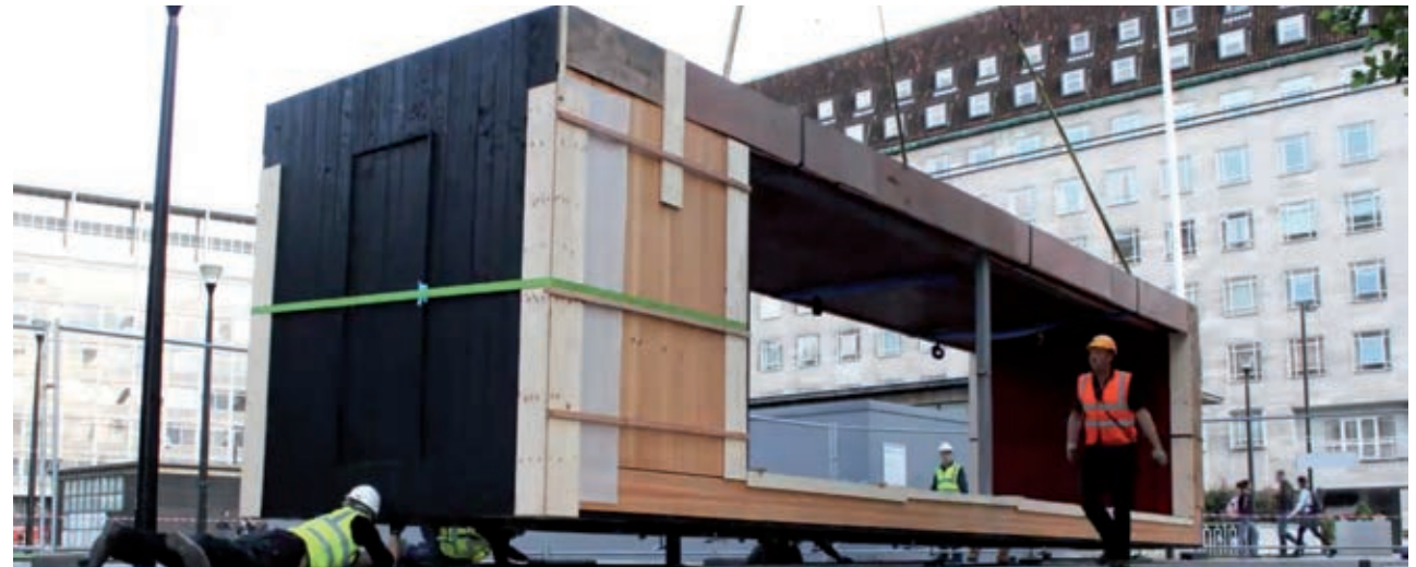
Fig. 18a-c Dresser under construction
